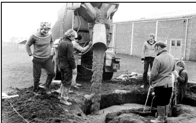
Working on the foundations of the observatory
